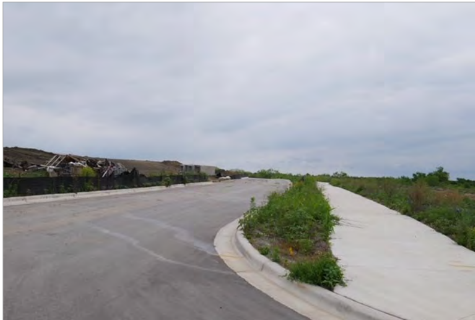
Liberty Bell Boulevard Looking North
